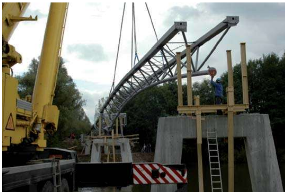
Lifting the 36 m span
