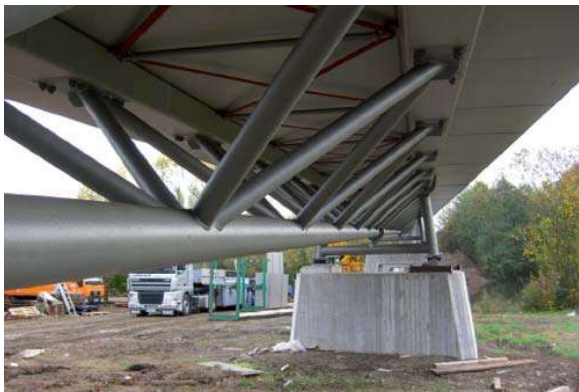
Superstructure soffit with slabs on top
