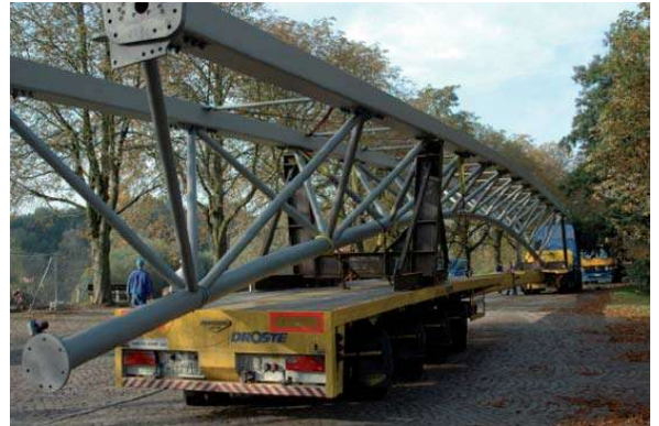
Lattice trusses with UHPC top chords
