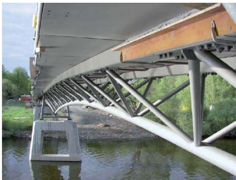
View of the fresh bond between top chord and carriageway slab
