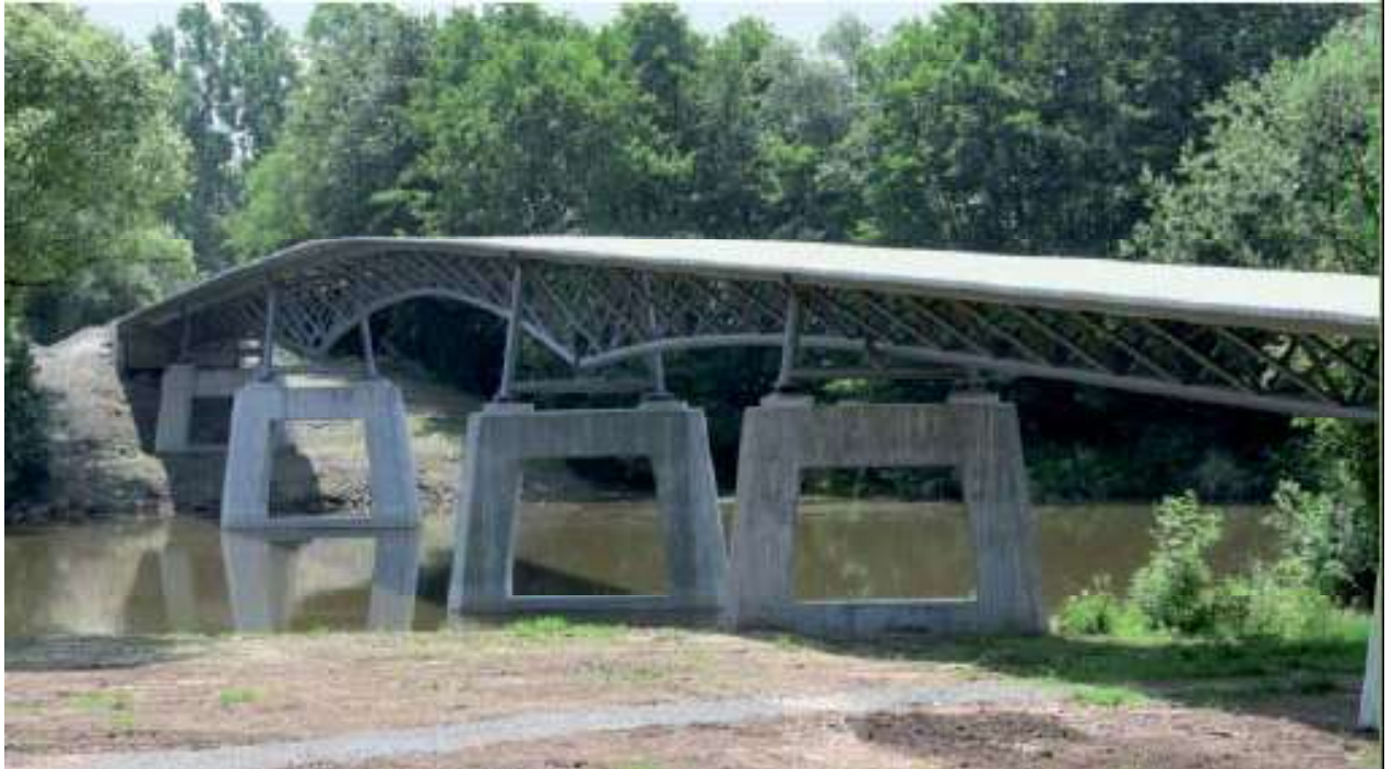
Gärtnerplatz Bridge shortly before completion
