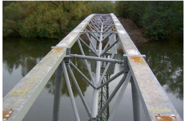
Lattice truss installed
