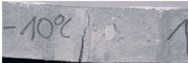
Typical cracking adjacent to the bond in the test slab concrete
